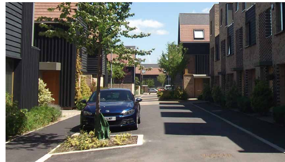
Shared surface lane with parking and street trees
