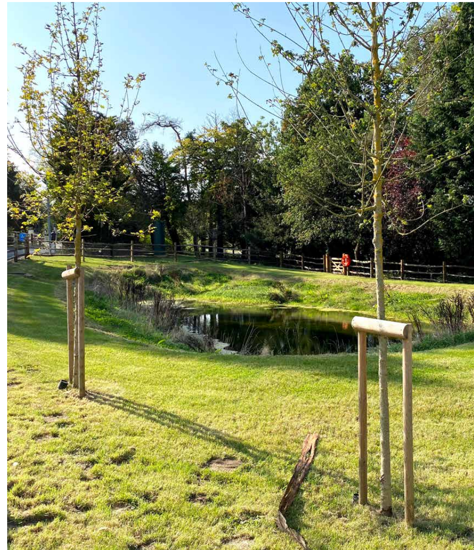
Landscaped attenuation basin
